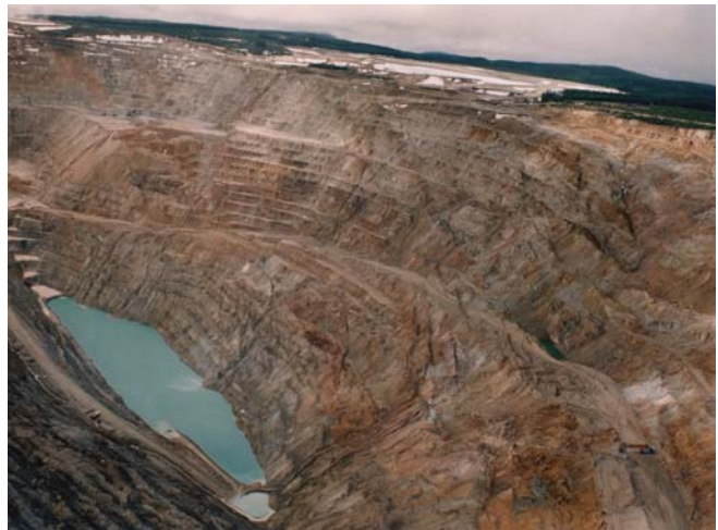
Figure 5 - Case History # 4, - Toppling Instability
