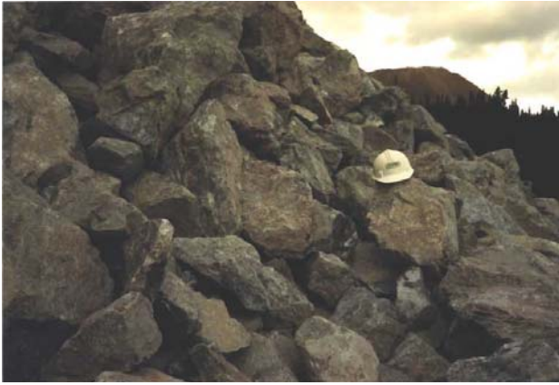
Figure 5 Rock 10m above toe (Golder 1987)
